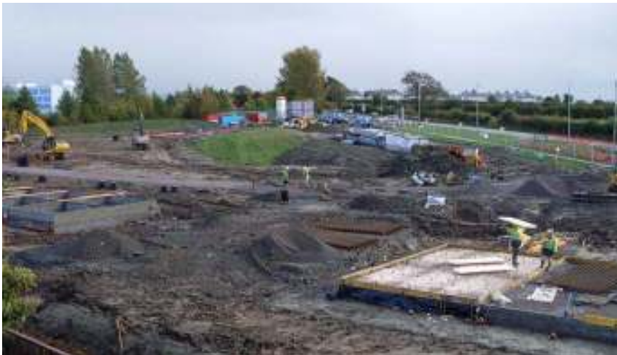
Our new build development site off Castlehill Road
